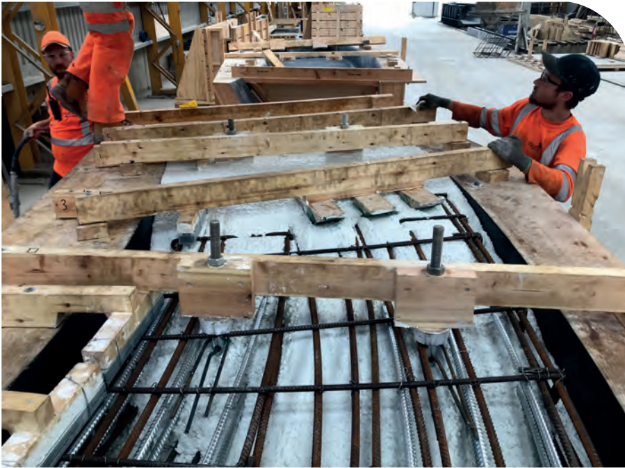
LEFT: During casting of pendentive 'wings'.
