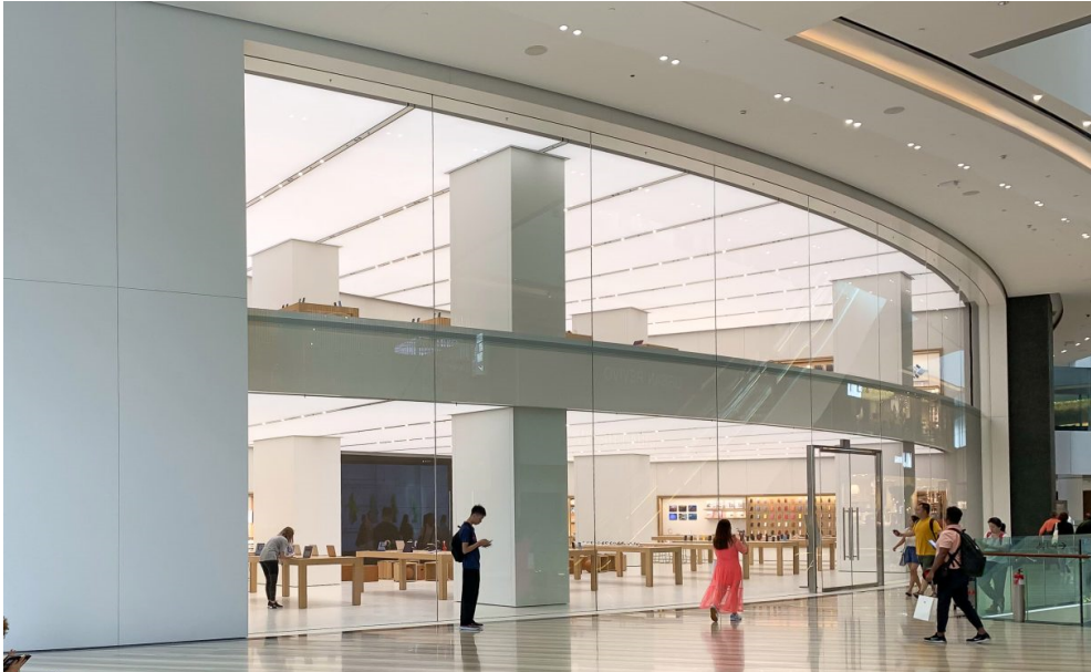
Fig. 5 Thermally toughened warm-bent (lamination-bent) glass fabricated by Sedak. Singapore Jewel Apple Store. Architects: Woods Bagot HK | Structural Engineers: Eckersley O'Callaghan | Contractor: Seele Austria
