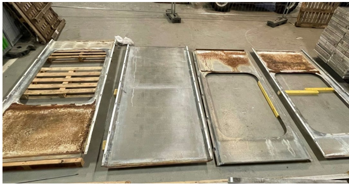
Dismantled aluminium facade elements
