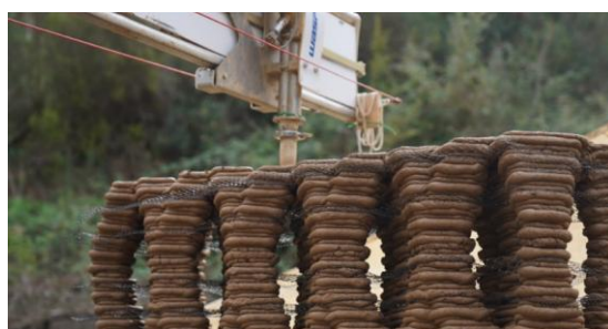
Figure 15: Test print of the clay walls completed by IAAC
